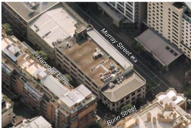
Figure 56 – oblique aerial of 55-65 Murray Street
