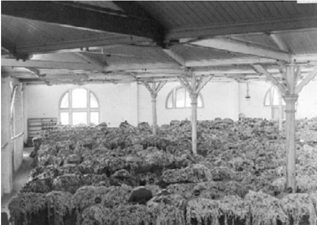
Top floor interior of 28-48 Wattle Street (Winchcombe Carson Ltd) c. 1901 Source: Museums of History NSW, NRS-4481-3-[7/16280]-St1455
