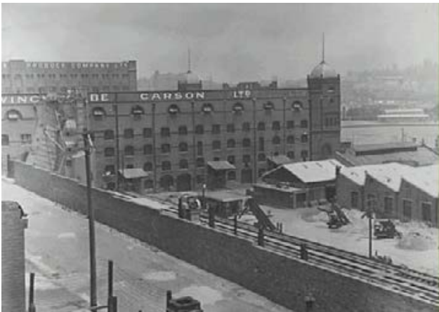
Wincombe Carson Ltd and Wentworth Park in background, 2/12/1957 Source: Sydney City Archives, SRC13690
