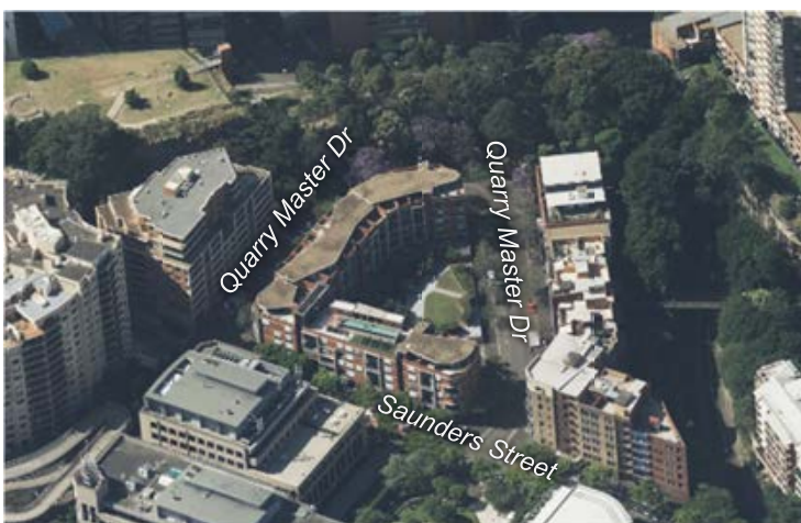
Figure 74 – oblique aerial of 26-38 Saunders Street
