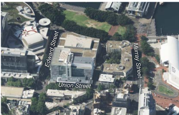
Figure 37 – oblique aerial of 1-27 Murray Street
