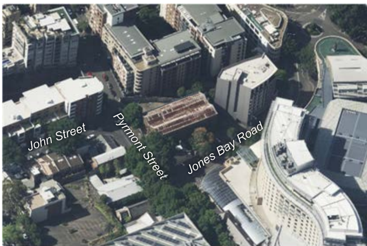
Figure 102 – oblique aerial of 12 Pymont Street
